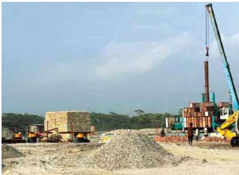
Ongoing construction work of upcoming Patuakhali EPZ
