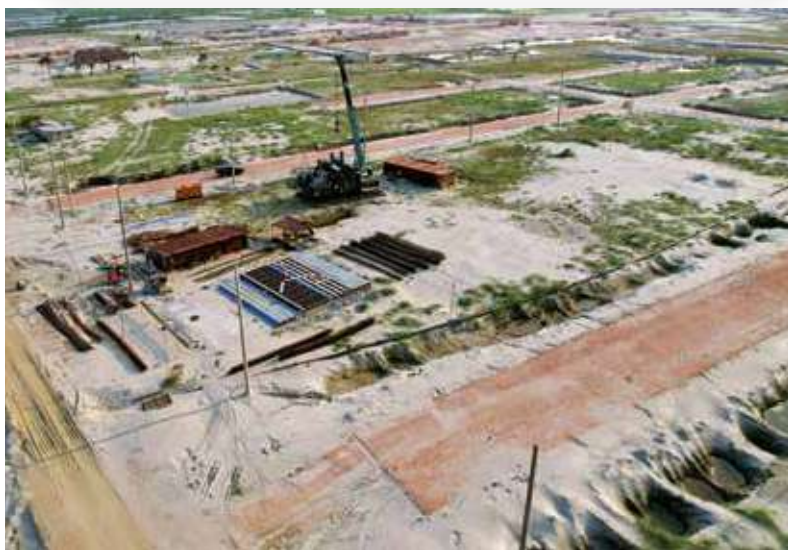
Construction work of upcoming Jashore EPZ progressing rapidly
